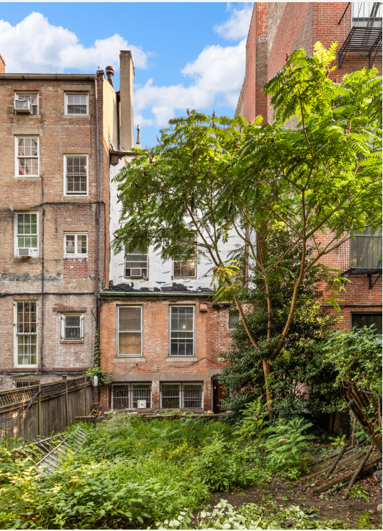
AS-IS REAR FACADE
